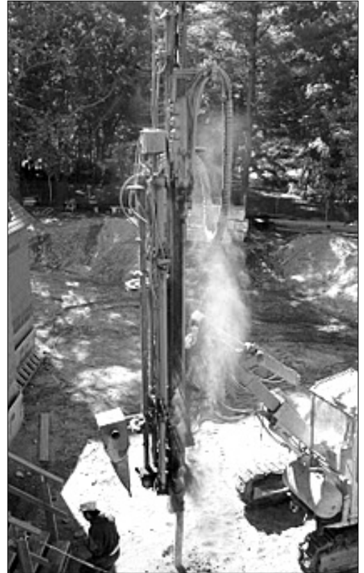
Drilling the geothermal wells
